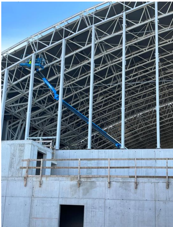
The Genie boom's articulating jib made it the ideal machine for steel work in confined spaces
