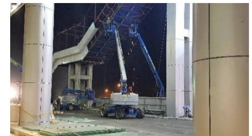
Mechanical & Engineering work
