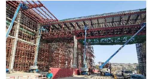
Genie boom's outreach capability allows it to be deployed off road
