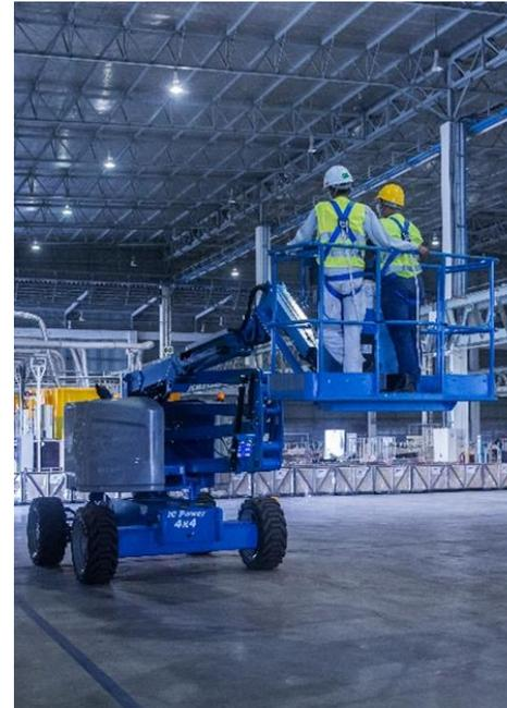
Replacing lamps at 12 m high with Genie Z-45/25J RT boom lift
