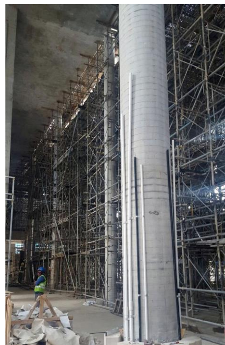
BEFORE – With 100% Scaffolds
