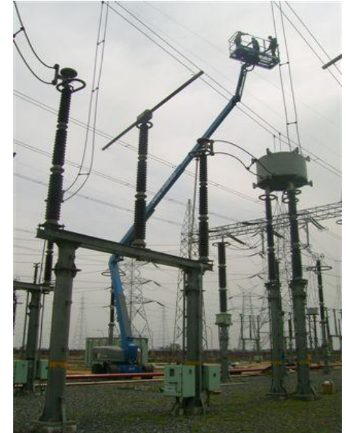
Genie booms' platform can go up and over the cable lines
